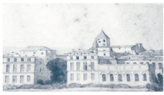
2 ème phase de construction / 2nd phase of construction
